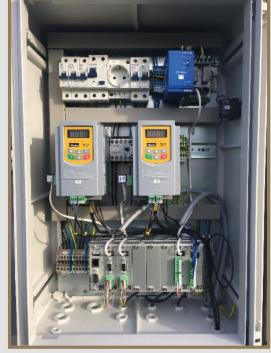
The antenna control unit is designed for IP-based control from a PC running a graphic user interface compatible with standard web browsers. The control GUI displays all the information required to set and maintain azimuth, elevation and polarization, including current position and target position plus a database of potential accessible satellites.
